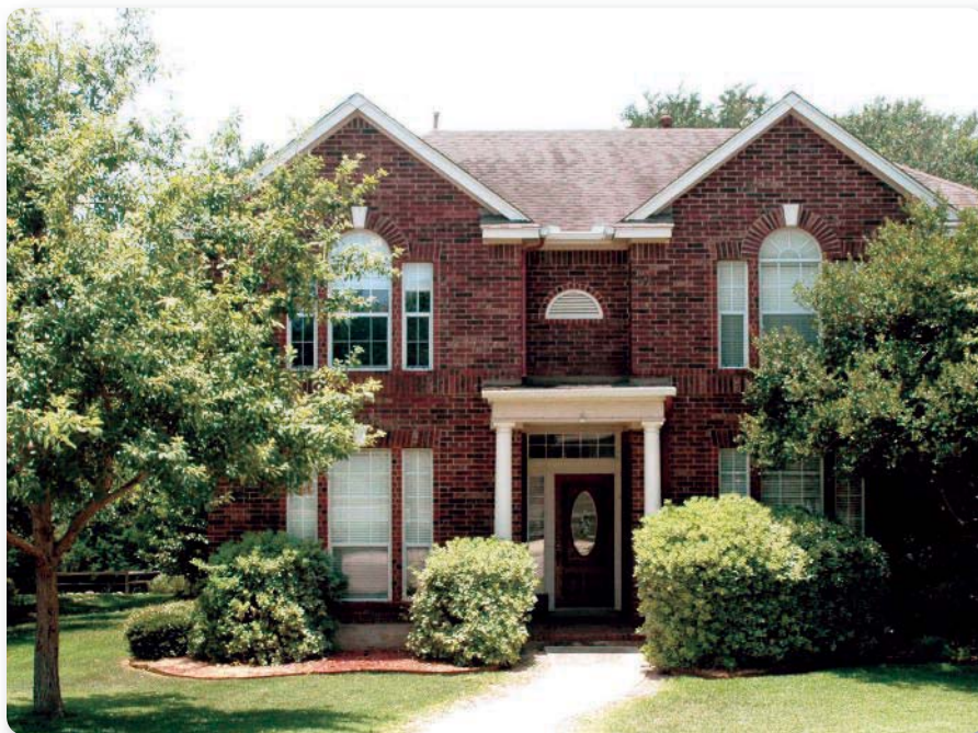
For every home, the correct amount of heating and cooling must be calculated, not guessed. General Air came to the rescue for this home that had too much of both.
