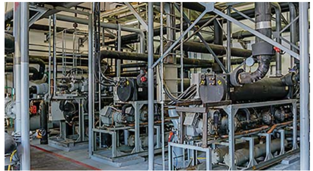
Refrigeration rack installation. Photo credit: Climate Pros.
