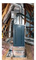
Mitsubishi intelli-HEAT™ (shown here installed atop a furnace) works seamlessly with existing furnaces.
