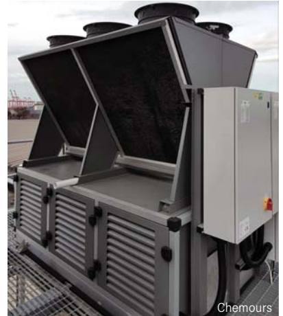
ASDA's Bootle supermarket initially deployed a Trans-critical R-744 CO 2 booster system during the 2007 reconstruction, comprised of two centralised medium temperature racks and one low temperature rack with one common remote gas cooler.
